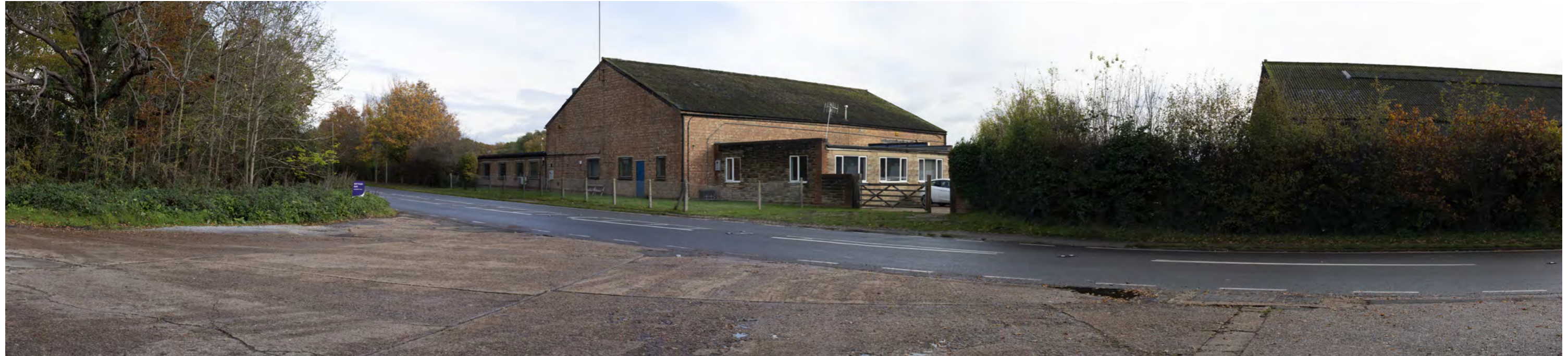
Photograph Viewpoint 5: A319 at entrance to Chobham Business Centre
