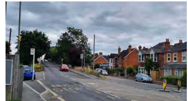
Figure 77. Frimley Road/ Moorlands Road / Oakley Road junction requires improvements to accommodate the proposed priority crossing
