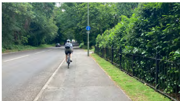
Figure 64. Existing shared use path along the A30
