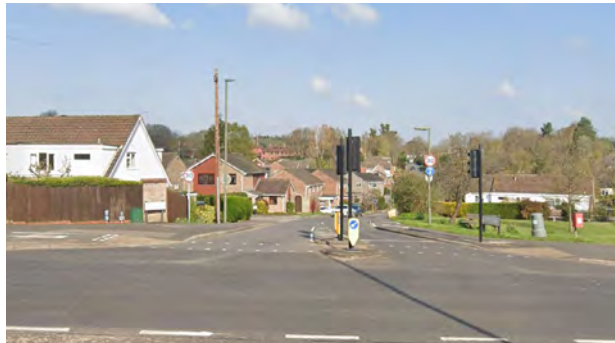
Figure 127. London Road (A30) signalised junction with Yaverland Drive lacks dedicated pedestrian phase on the minor road arm. (image: Google StreetView)
