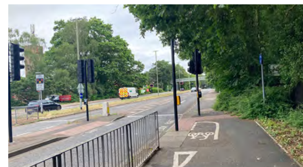
Figure 67. Improvements to the existing cycle facilities along the A30. New facilities would allow for a continuous cycle route to link Camberley and Bagshot.
