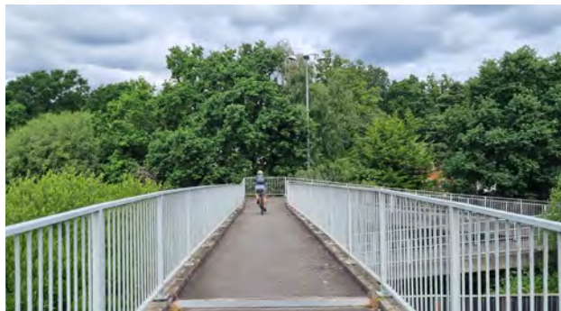
Figure 82. M3 footbridge is narrow (approx. 2.2m width) and widening will be required if the pedestrian and cycle flows increase.
