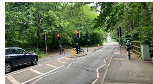
Figure 65. Existing crossings on the A30 to be retained and upgraded to toucan crossings to accommodate cyclists
