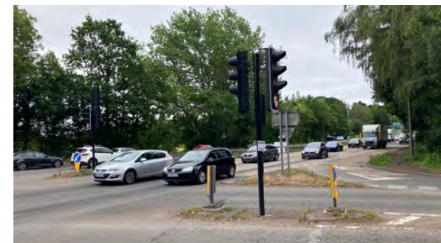
Figure 93. New Road/Bagshot Bypass junction does not provide crossings for pedestrians and cyclists
