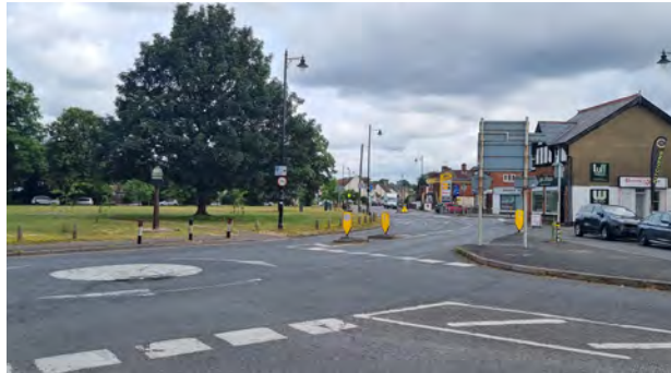
Figure 89. Changes to Frimley Green Road/ Sturt Road/ Guildford Road roundabout to a priority junction are required to increase the space for pedestrians and cyclists, introduce priority crossing and tidy vehicular movements.
