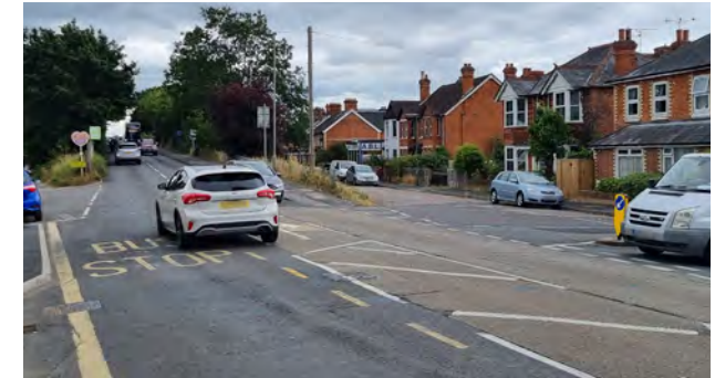
Figure 105. Minimal pedestrian provision at Frimley Road junction with Moorlands Road and Oakley Road.
