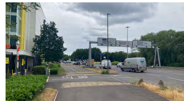
Figure 72. Existing cycle facilities and crossings at The Meadows Roundabout.
