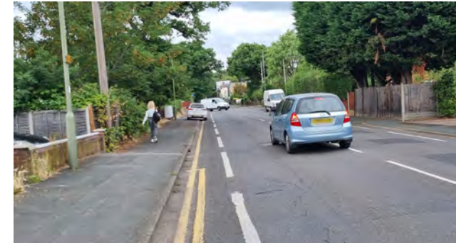
Figure 76. Existing advisory cycle lanes on the north extent of Frimley Road to be upgraded to segregated cycle tracks.
