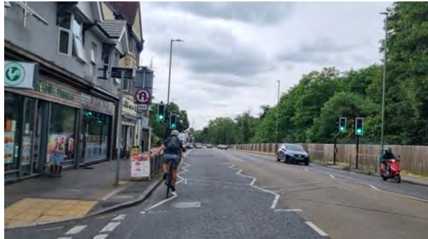
Figure 104. London Road existing signal controlled crossing near Victoria Avenue junction.
