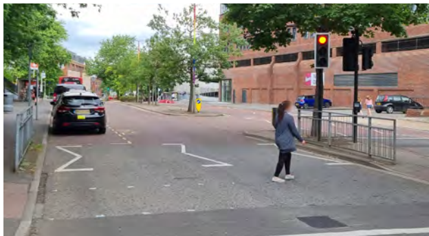
Figure 106. Pembroke Broadway signal controlled crossing near the railway station to be upgraded to a toucan with removed guard railing.
