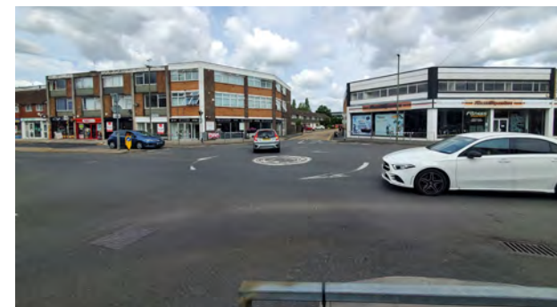
Figure 112. Frimley High Street / Hale Way / Cedar Lane junction. Roundabout provides access to Waitrose car park. Car dominance with guardrail, convoluted and constrained pedestrian crossings.
