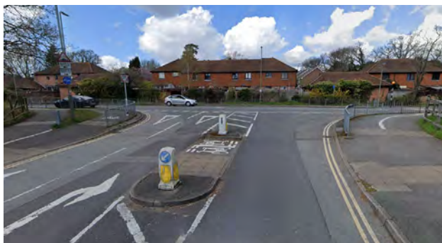
Figure 113. Tomlinscote Way junction with Chobham Road has wide junction bellmouth with multiple exit lanes. (image: Google StreetView)
